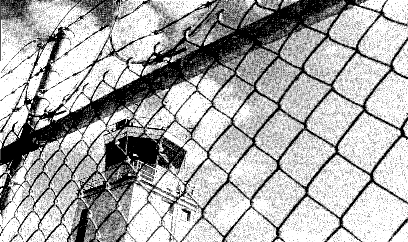
The control tower at the former U.S. Marine Corps Air Station, strategically located only a few miles from California's coast. Photo: Control Tower by Nazgol Zandyazdani
